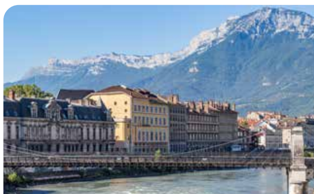
Saint Laurent footbridge and quays © F. Lucas
