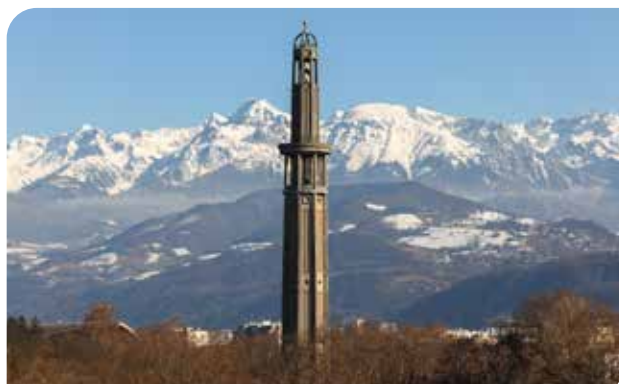
Perret Tower © City of Grenoble
