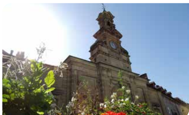
Saint-Pierre Gate, Pontarlier ©Philippe Ancelot
